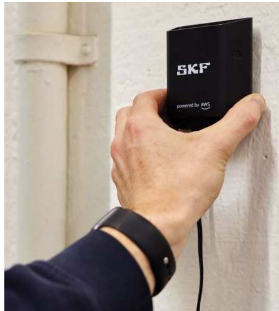
Physically installing gateway
